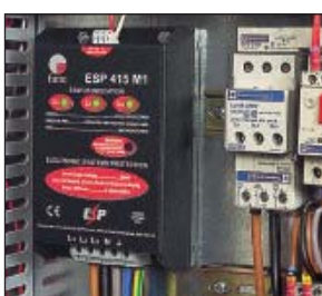
ESP 415 M1 installed within a control panel on the mains input to protect the panel's control systems. Note the remote indication connection (top of protector)
