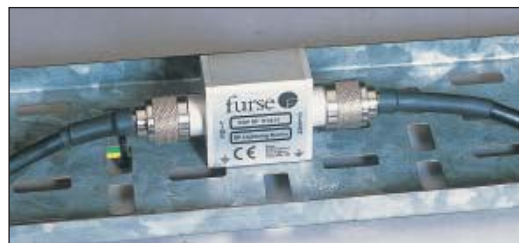
ESP RF 111A11 installed on a coaxial cable running between an antenna and an RF receiver. Note the earth lead (behind the cable tray) attached to the mounting fixture
