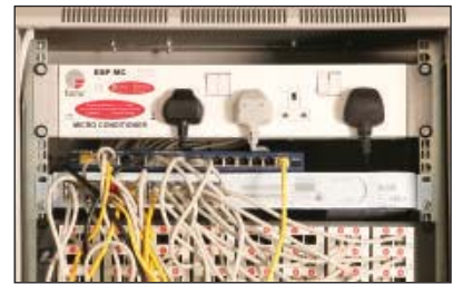
ESP MC installed within a network rack, protecting the externally-fed network switch
